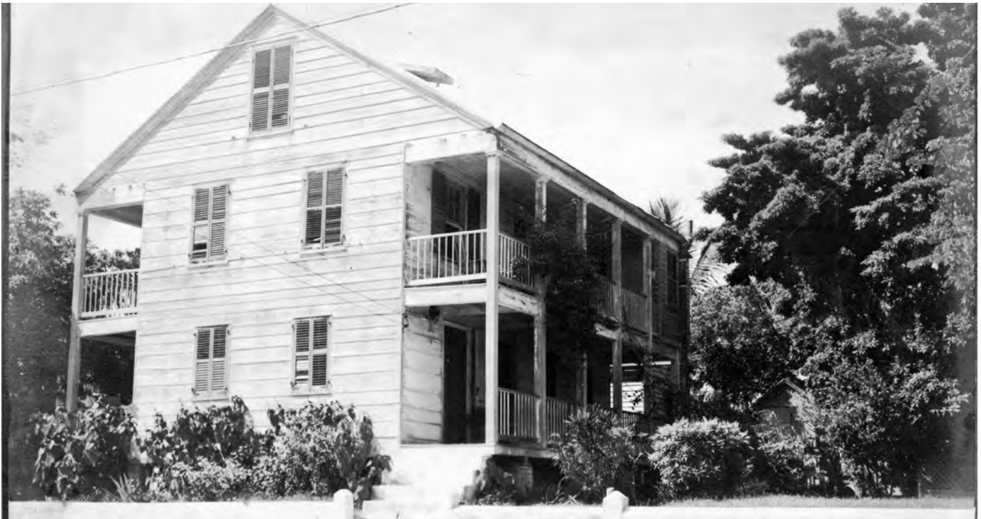
The house at 408 William Street that Tuggy Roberts moved from the Green Turtle Cay, Photo credit: Monroe County Library.
