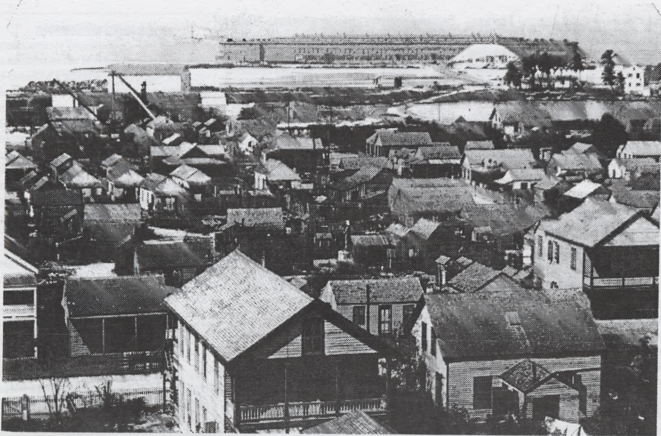
Fort Taylor from the Key West Lighthouse. To the left of the Fort is the USS Maine. Photo credit: Monroe County Library.
