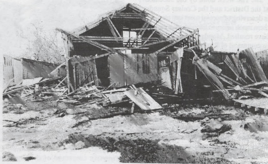
A building wrecked by the hurricane. Photo credit: Monroe County Library.
