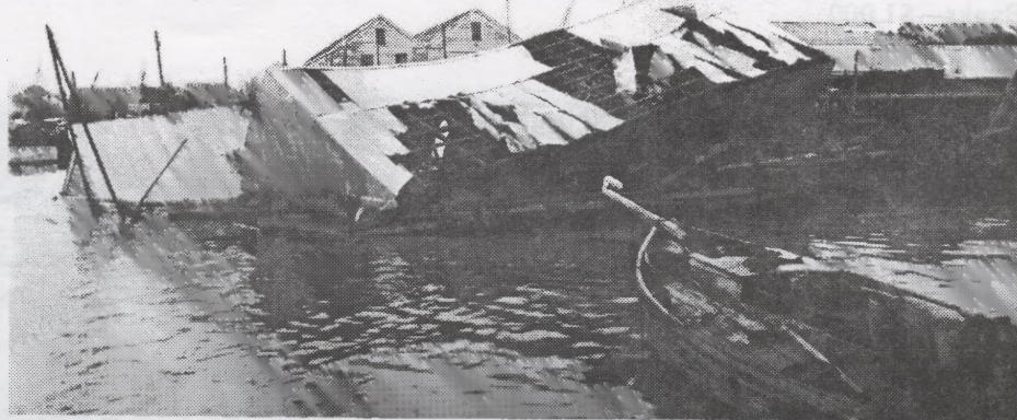
Buildings on the waterfront destroyed by the hurricane. Photo credit: Monroe County Library.
