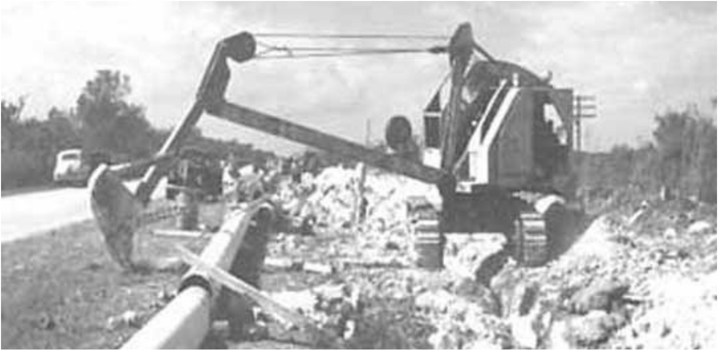
Trench for the water pipeline. Photo credit: Monroe County Library.
