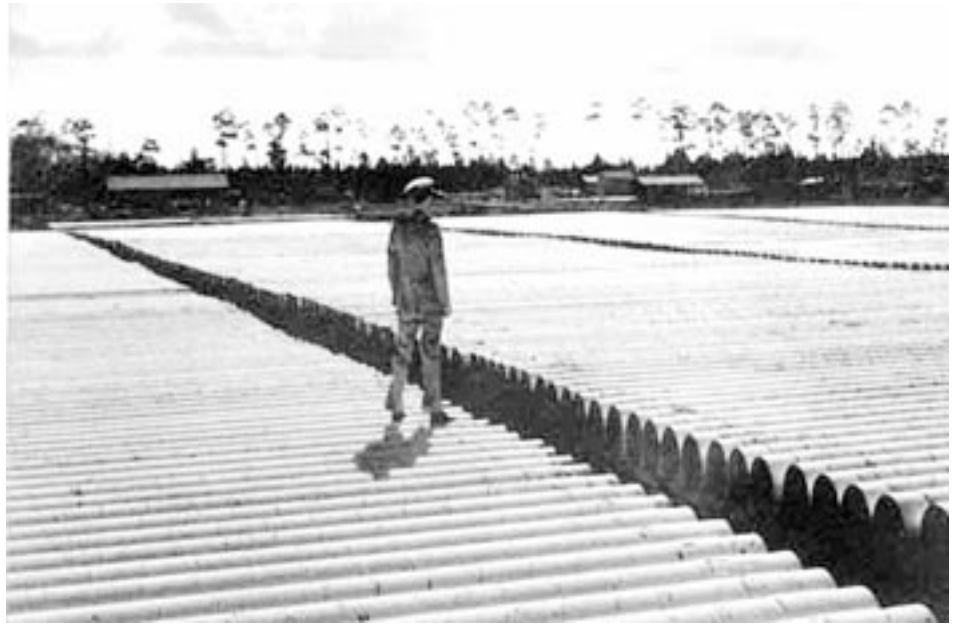
Pipes at Florida City for the water pipeline. Photo credit: Monroe County Library.
