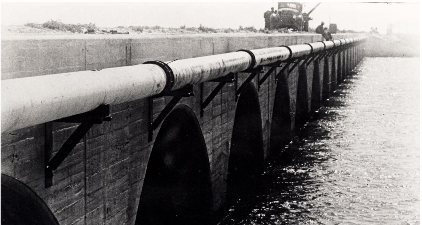
Water pipeline installed on a railroad bridge. Photo credit: Monroe County Library.
