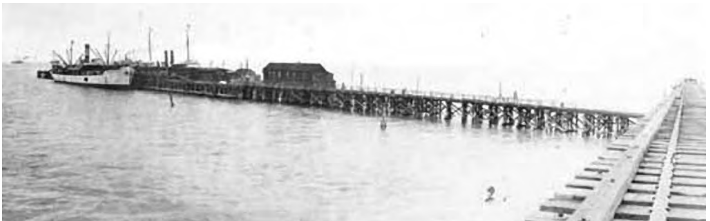
: The Knights Key Dock as seen from the Knights Key Bridge. A free-standing wooden platform the length of two football fields, the dock was connected to Knights Key by a temporary trestle. The Knights Key Bridge, which was built over the trestle, was designed with sufficient clearance to allow trains to continue accessing the dock. Bottom: The trestle emerges on the north side of the Knights Key Bridge and curves around to Knights Key in the distance. Photo credit: State of Florida Photographic Archives.
