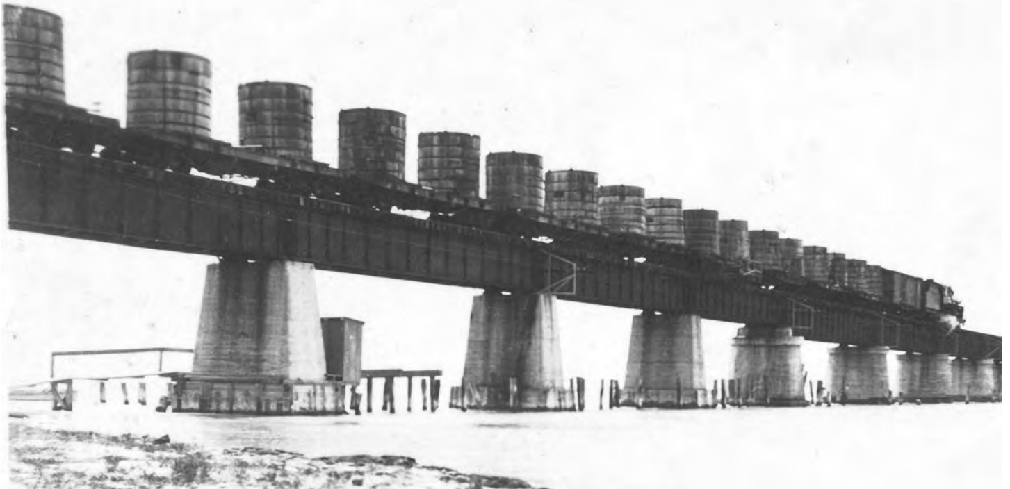
Potable water for Pigeon Key and other FEC Railway installations including the station and yard at Key West was delivered from the mainland in cypress water tanks carried aboard flatcars. At Pigeon Key the water was transferred to elevated tanks located adjacent to the track. The latter were attached to concrete piers so that they hung over the water on the east and west sides of the island. Part of the west outhouse/shower is visible above on the leftmost pier. Photo credit: State of Florida Photographic Archives.
