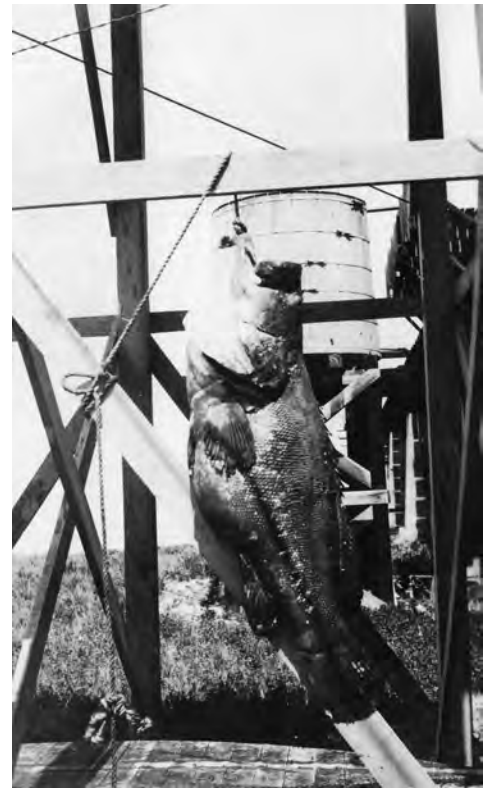
Raleigh Hines and others often fished in the adjacent waters bringing in catches such as this jewfish (now known as goliath grouper). The elevated cypress tanks in the background held fresh water delivered by train from the mainland. Photo credit: Marshall L. Brewton Jr.
