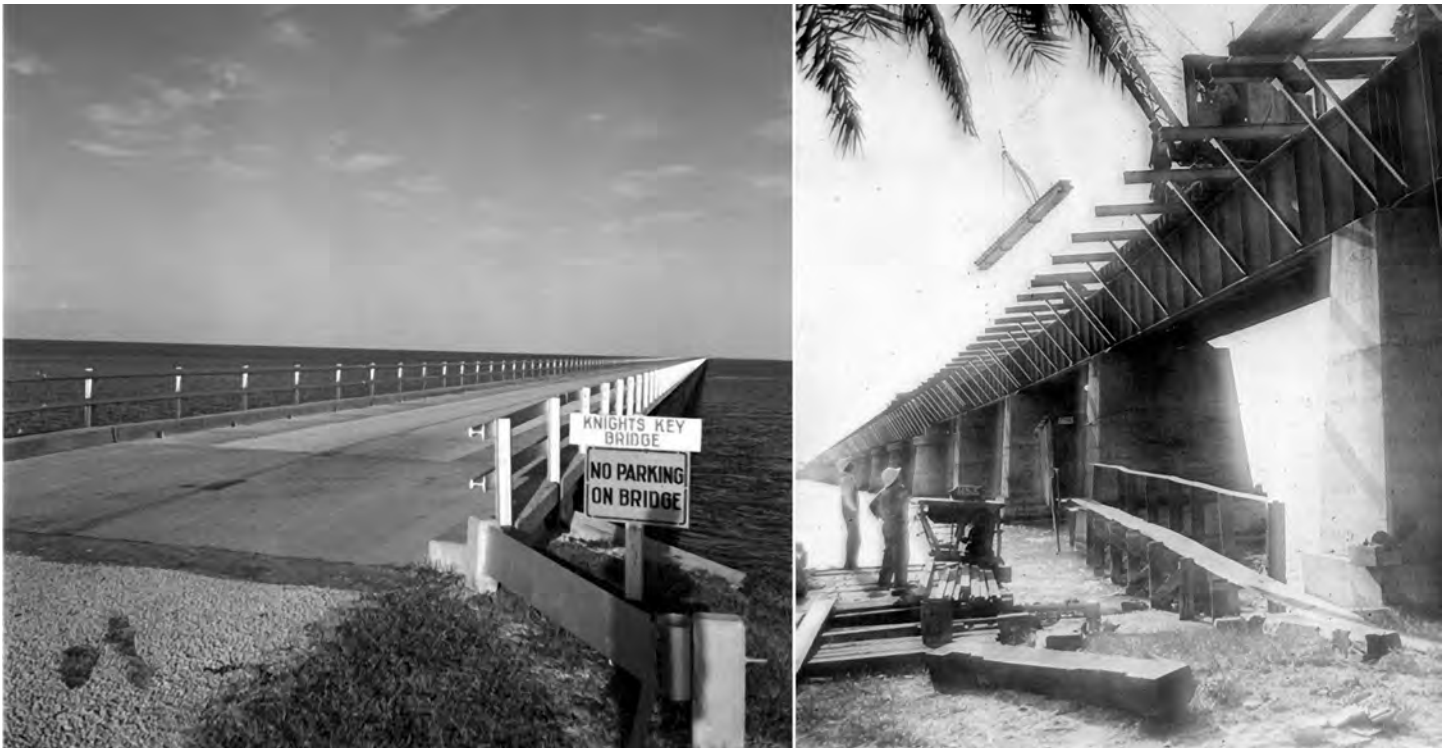
In 1937 railroad bridges were modified to make a continuous highway to Key West. Above right: The Pigeon Key Bridge is widened to accommodate two lanes of automotive traffic by placing steel beams across the girders. Left: Entrance to the Knights Key Bridge after modification. Forty miles of rails salvaged from the defunct railroad were used make the guardrails for the bridge between Knights Key and Little Duck Key. Photo credit: State of Florida Photographic Archives.
